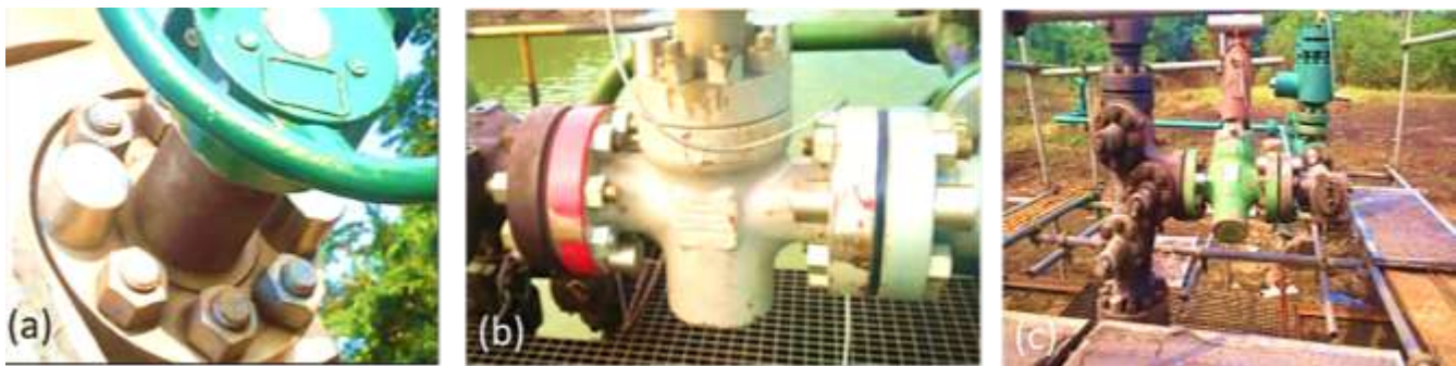
Figure 4: Sureguard® (a) installed on flanges (b) and wellhead (c) in remote locations (BGT, 2018).
